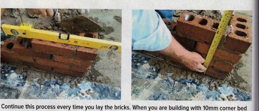
joints, if you are using 65mm bricks, set your Mortar Joint Gauge to 75mm to establish the mortar thickness. them on site we found that we couldn't securely clamp the Gauge to the spirit level. That meant going back to the
